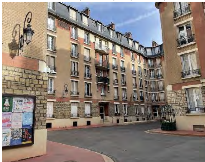
REHABILITATION DE LA RESIDENCE BERTHELOT
